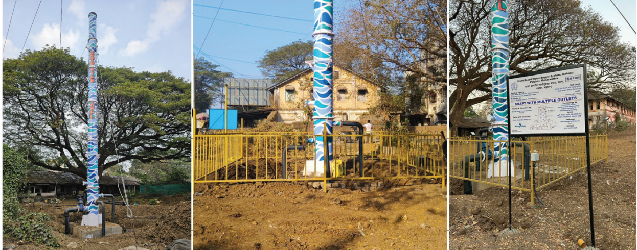
Figure 43: Shafts installed at Dahanu water supply zone
