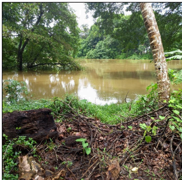
Figure 54 : Lack of side wall
