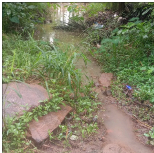
Figure 49: Absence of Culvert
