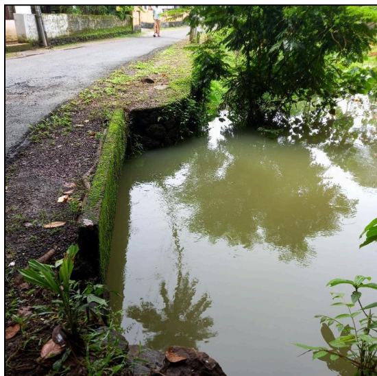
Figure 56: Insufficient Culvert
