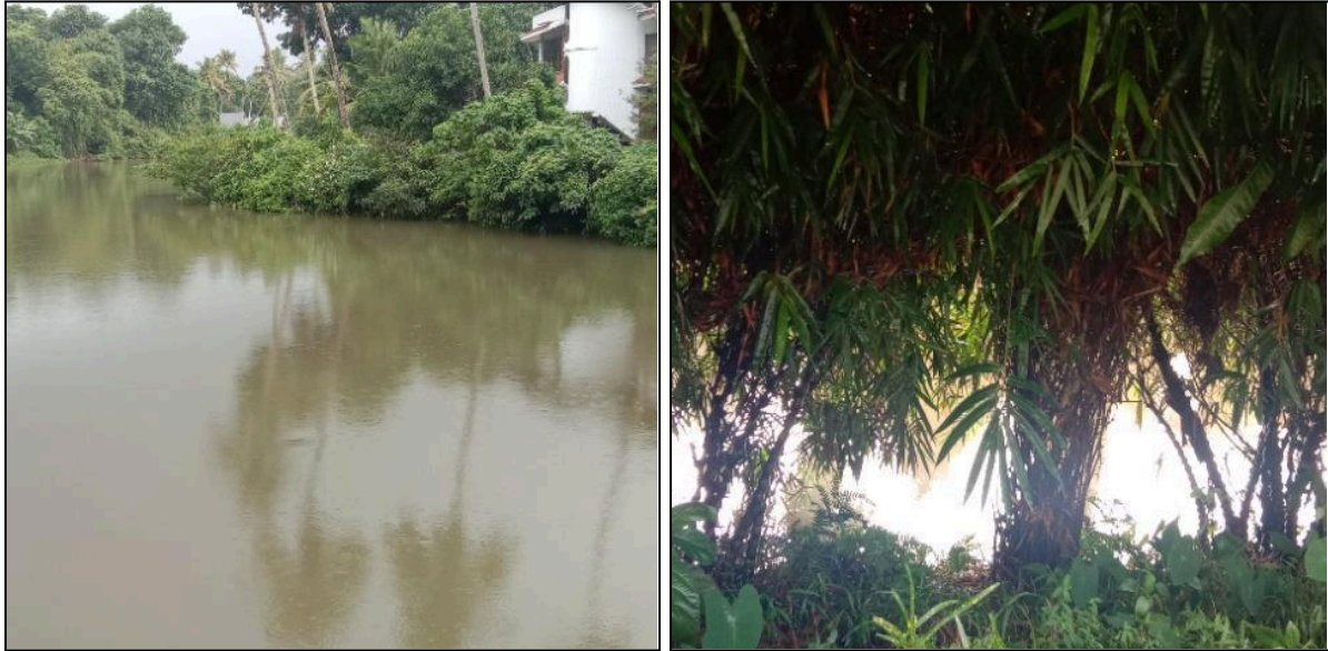
Figure 43: Encroachment due to Vegetation
