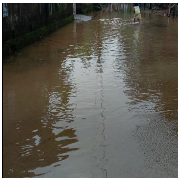
Figure 39: Absence of Drainage Facility
